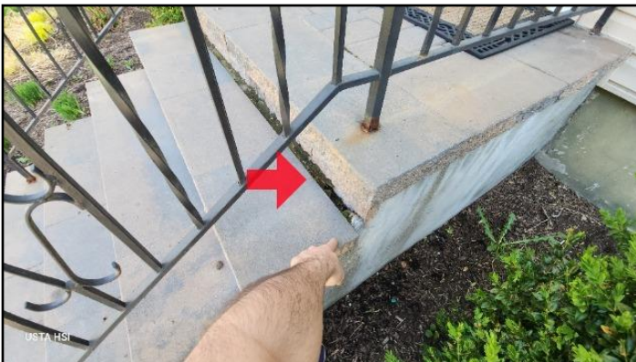
Missing or deteriorated mortar was observed...
