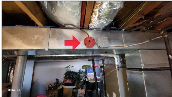
Oil burner shut off observed, no oil tank obs
