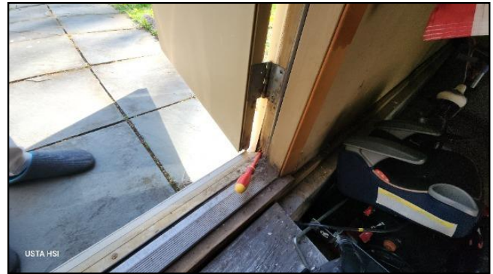
Areas of rot or decay were observed on the...
