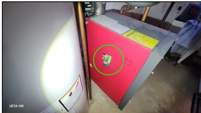
The temperature and pressure relief (TPR)...
