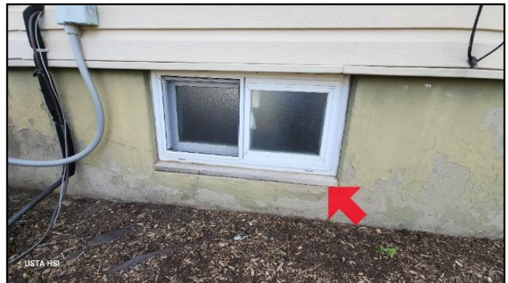
Exterior window jambs and trim surfaces sho...
