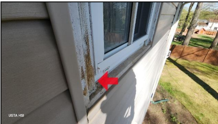
Exterior window jambs and trim surfaces sho...
