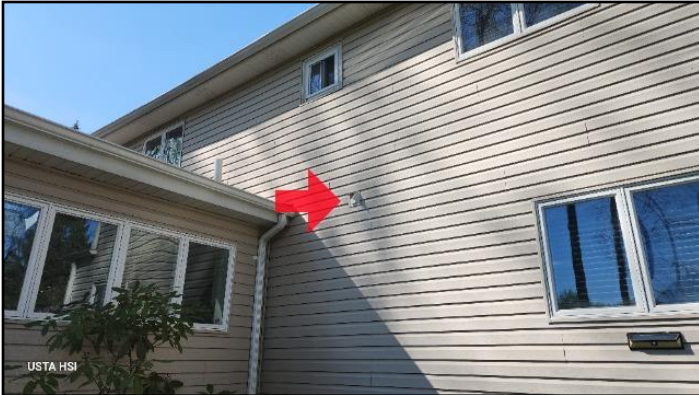
A damaged vent cover was observed.
