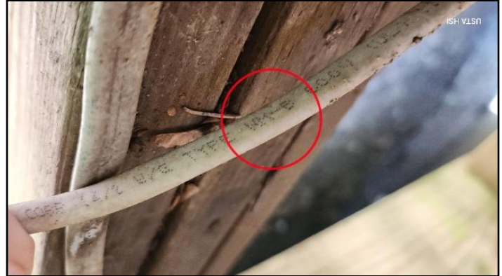
Electrical wiring observed that is not rat...
