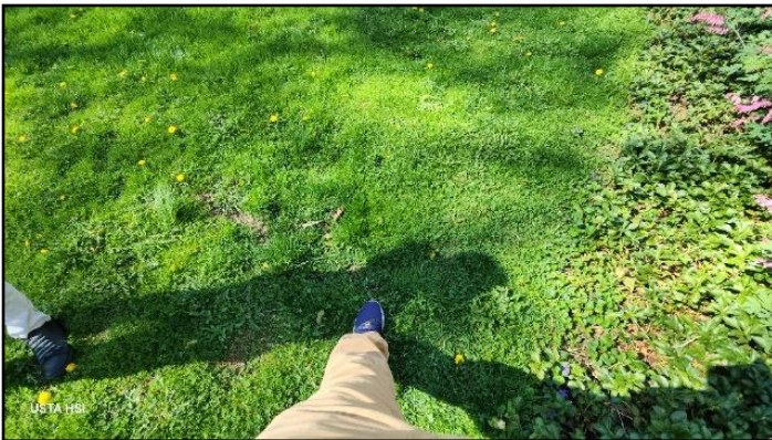
Depressions were observed in the ground...
