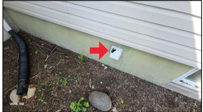
A damaged vent cover was observed.
