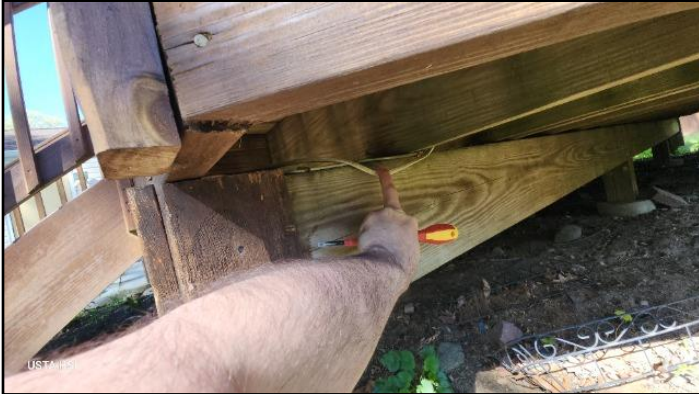
Electrical wiring observed that is not rat...
