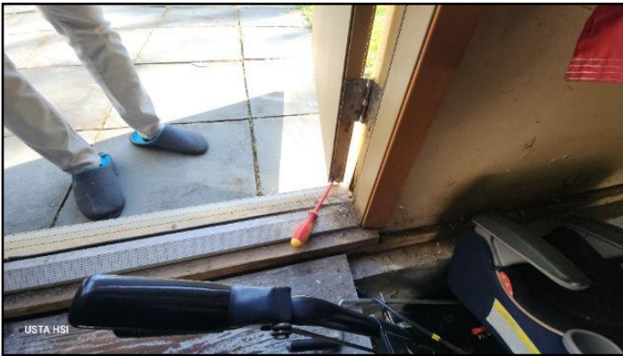
Areas of rot or decay were observed on the...
