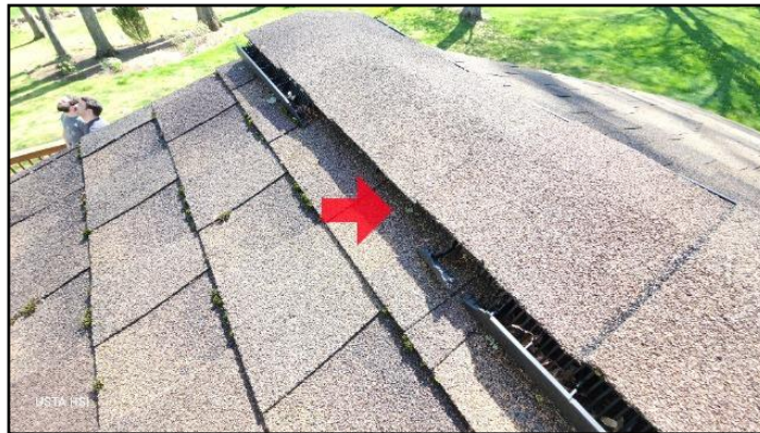
Sections of the ridge vent screening were...
